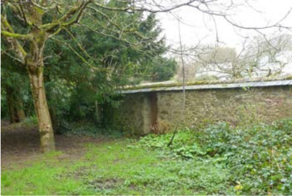
Grove Hill kitchen garden walls – stone and some cobb (poor condition and at risk).
