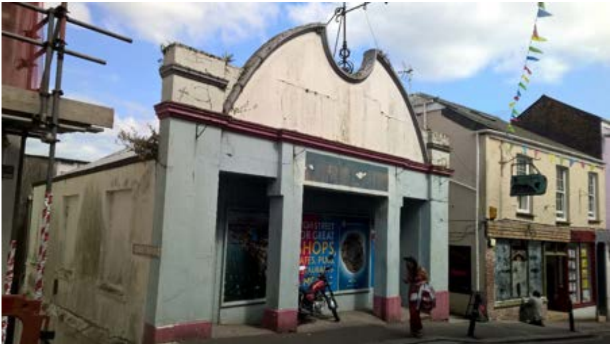
Condition in 2018. Nothing maintained since Camellia Designs left, and considerable deterioration to the parapet, with vegetation growing, cracks appearing and damp evident. There is concern also at the condition of the decorative ironwork.
