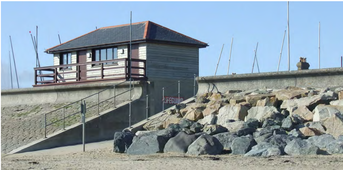
Above: Defences at Marazion – a concrete wave return seawall is fronted by both rock and concrete sloped revetments
