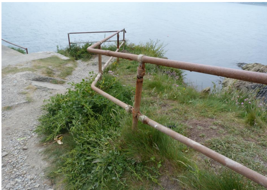
Fig 10 CAR PARK GALVANIZED RAILINGS - TO BE REPLACED
