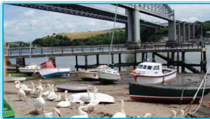
8 Saltash and the Tamar Bridge
